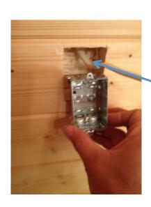
Interior divisional walls are pre-drilled with electrical chases during production. Wiring is installed during assembly and surface mounted or countersunk electrical outlets are used.
